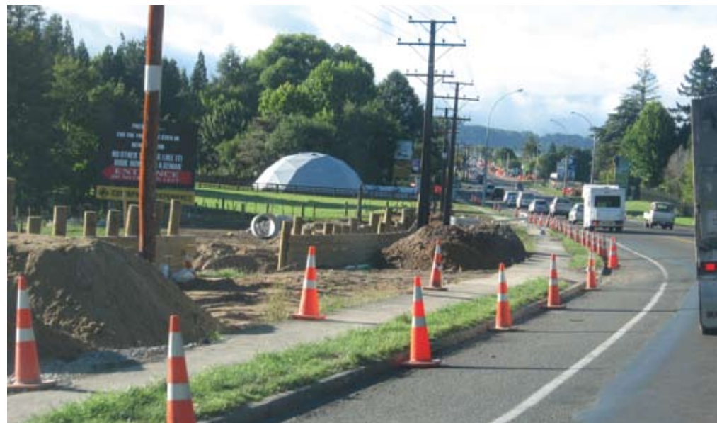
Fairy Springs Road before
